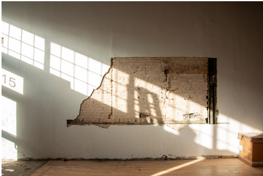
Exposed brick and finished hardwood floors
